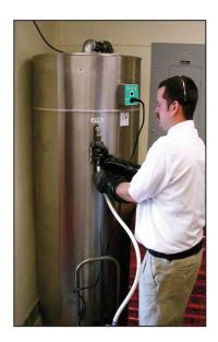
**4**. Remove the electrical cord from the heater and plug the cord into the motor on top of the caddy and into the receptacle on the storage tank control panel.
